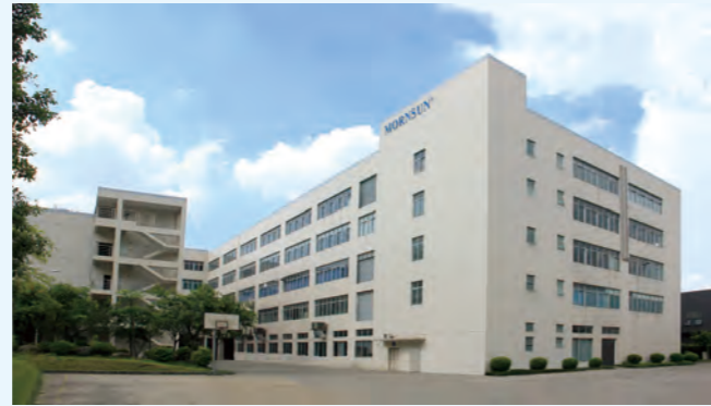
R&D Center in Guangzhou
